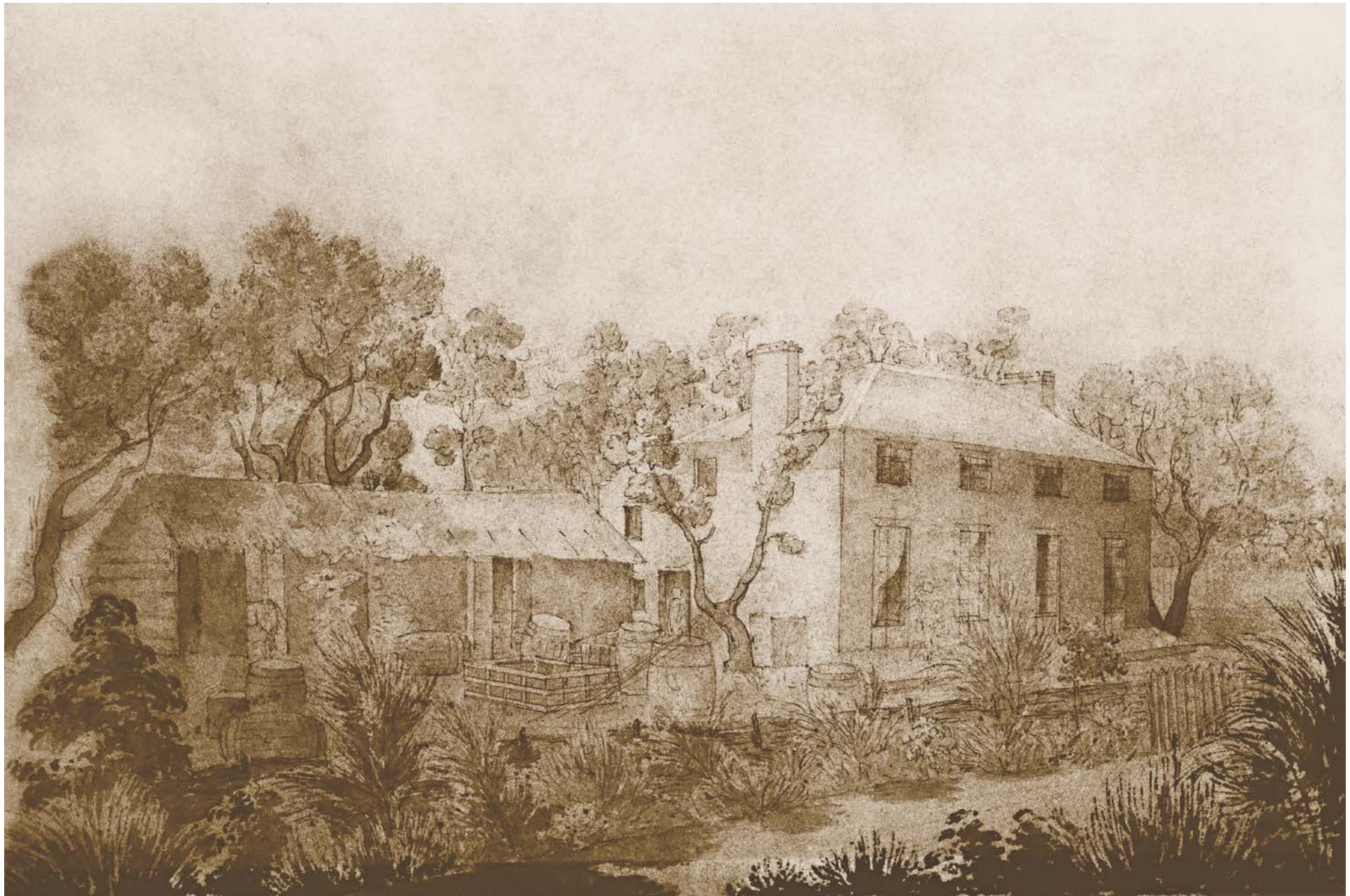
Colonial chaplain the Reverend Wittenoom's House in Perth drawn by his brother Charles Dirck Wittenoom whilst on a visit in the 1830s. Wittenoom and his sons had made the bricks from soil on the block and employed a bricklayer to build the house.
